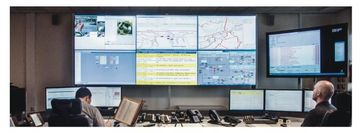
A Crestron TPS-6 touchscreen controller and remote KVM controls are installed on the main operators' console. This touchscreen controller enables the selection of a number of preset videowall configurations. The image processor allows any source image to appear at any size anywhere on the display.
